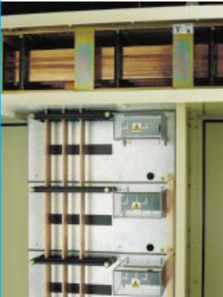
Fig. 1.7 The vertical MMX busbars showing Horizontal Master Frame
