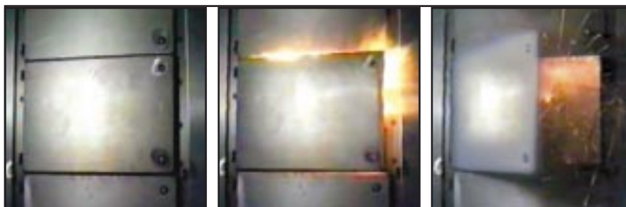
Photo 3 An MCCB on test at 50kA conditional. The breaker passed the test but the enclosure did not.
